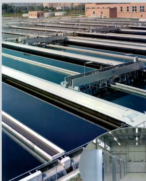
Depurazione acque reflue Waste water treatment
